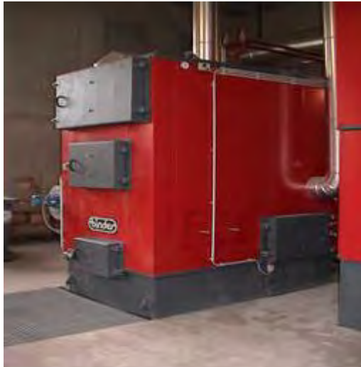
Photograph 3: Biomass Boiler
